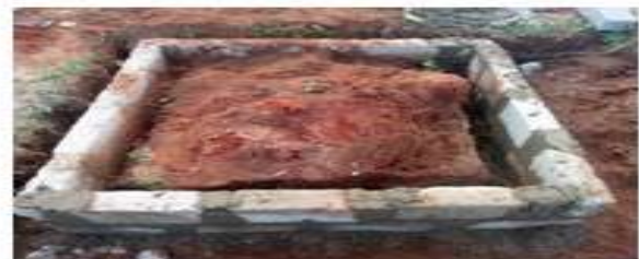
Plate 9: Erection of the foundation to cast the pedestal on which the sculptural work was mounted
