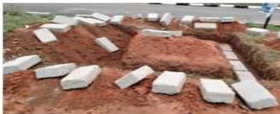
Plate 8: Provision of concrete blocks and commencement of foundation to cast the pedestal on which the sculptural work was mounted
