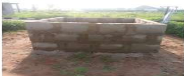
Plate 10: Erecting the concrete block casing for casting the pedestal on which the sculptural work was mounted.
