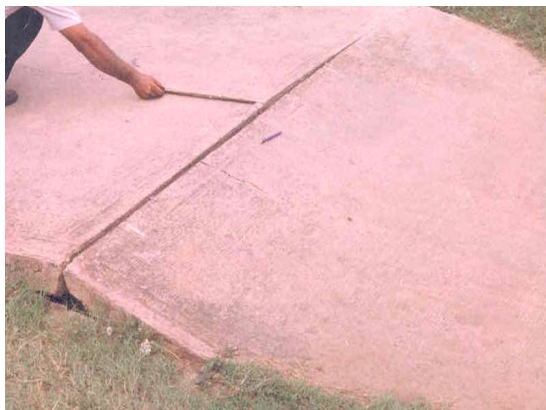
Photo 2. Blow-up of Concrete Slabs at Joint Photo 3. Transverse crack due to locked joint
