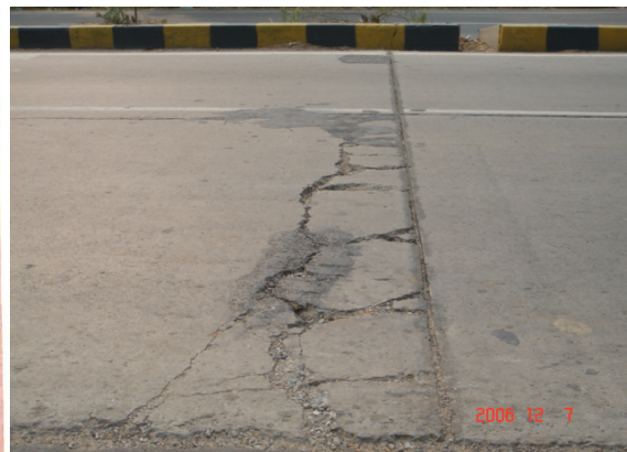
Photo 2. Blow-up of Concrete Slabs at Joint Photo 3. Transverse crack due to locked joint
