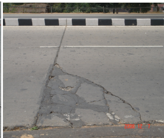
Photo 5. Corner Cracking
