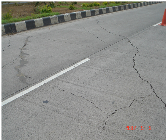
Photo 4, Settlement Cracking
